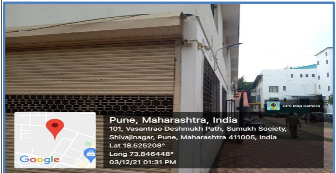
CCTV Installed at various area in campus
